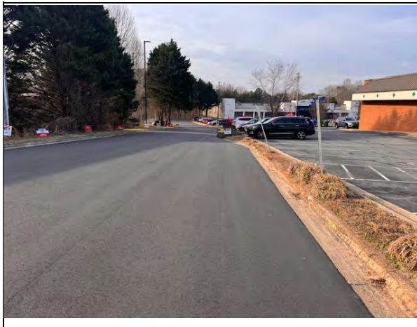
15. Land Acquired and w/in PUE facing Southwest Date of Photo - February 25, 2026
